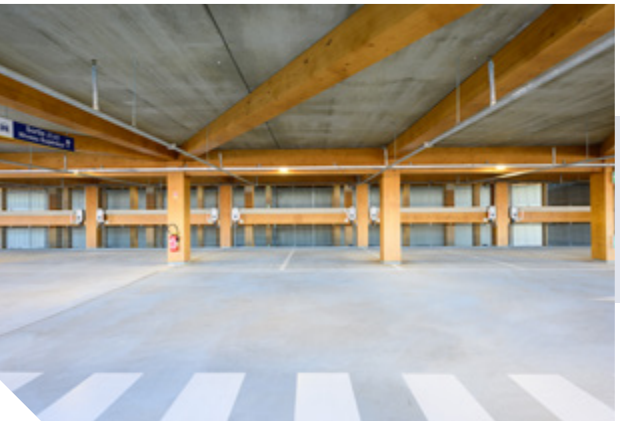
▲ Interparking Parking Station Saint-Jean Armagnac, Bordeaux (Frankrijk) PROJECTTYPE Parking ARCHITECT COSA Colboc Sachet architectures
