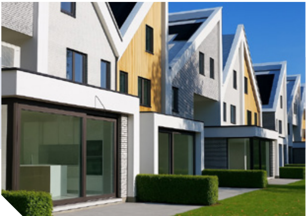
▲ Fenixco Menlo Park woningen, Sint-Amandsberg PROJECTTYPE Residentieel ARCHITECT A154 Architecten
