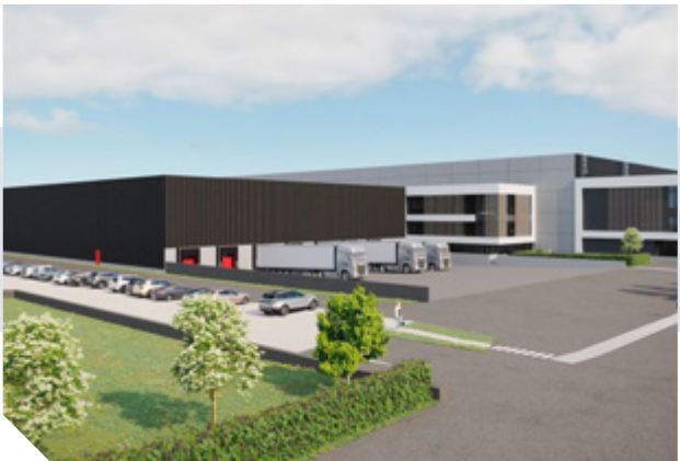
▲ Intervest Herstal Logistics, Herstal PROJECTTYPE Logistiek ARCHITECT Biemar & Biemar
